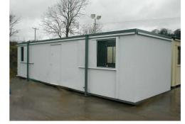
which is in turn supported on rolled steel channel skids extending the full length of the building. The whole floor is underdrawn with arson resistant galvanised sheet steel. The floor covering is a heavy-duty flexible sheet vinyl, with continuously welded joints, and is bonded to floorboards. Floors are designed to provide for a uniform floor loading of 2.5kn/m2. The floor can be insulated as an optional extra.
