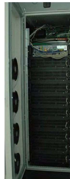
Figure 3-6: Inverter Phase Modules (3 per phase for a total of 9 modules) Installed in Power Stack
