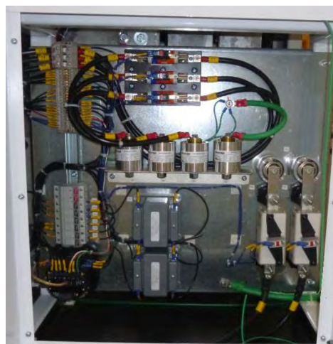
ACCESS COVER #4 / Strikesorbs, Current Transformers (CT-P1, CT-P2), Fuses (F2, 10F8, 10F9, 10F10, F11, F12, F17, F18, F19, 10F17, 10F18, 10F19, 10F20, 10F21), Power Meter (A4), Transformer (T1, T3, T4).
