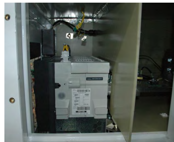
ACCESS COVER #4 / Circuit Breakers (CB2, CB3, CB4)
