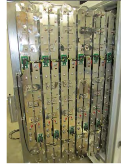
Figure 5-22a: GTB Filter Capacitor Panel
