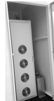
Figure 3-15: Evaporator Fans
