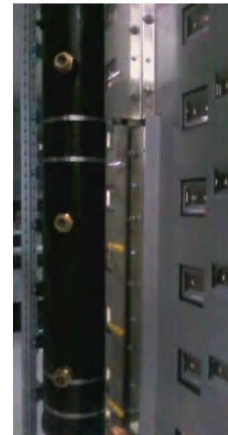
Figure 5-14: R134a Refrigerant Accumulator and Sight Glasses
