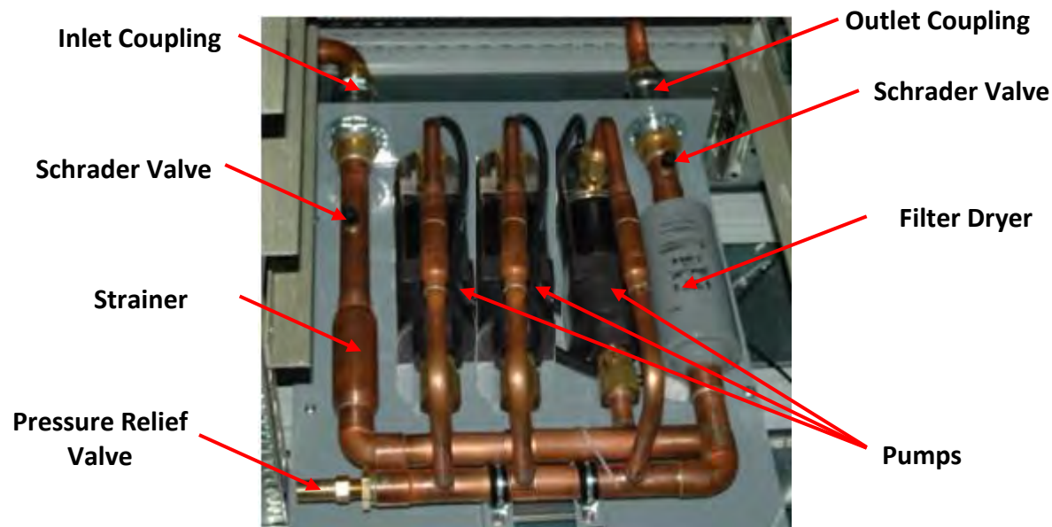
Figure 5-8: 3-pump assembly
