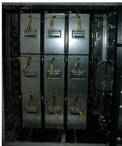
ACCESS COVER #3: AC Filter Inductors, Refrigerant Accumulator, Refrigerant Pump Module
