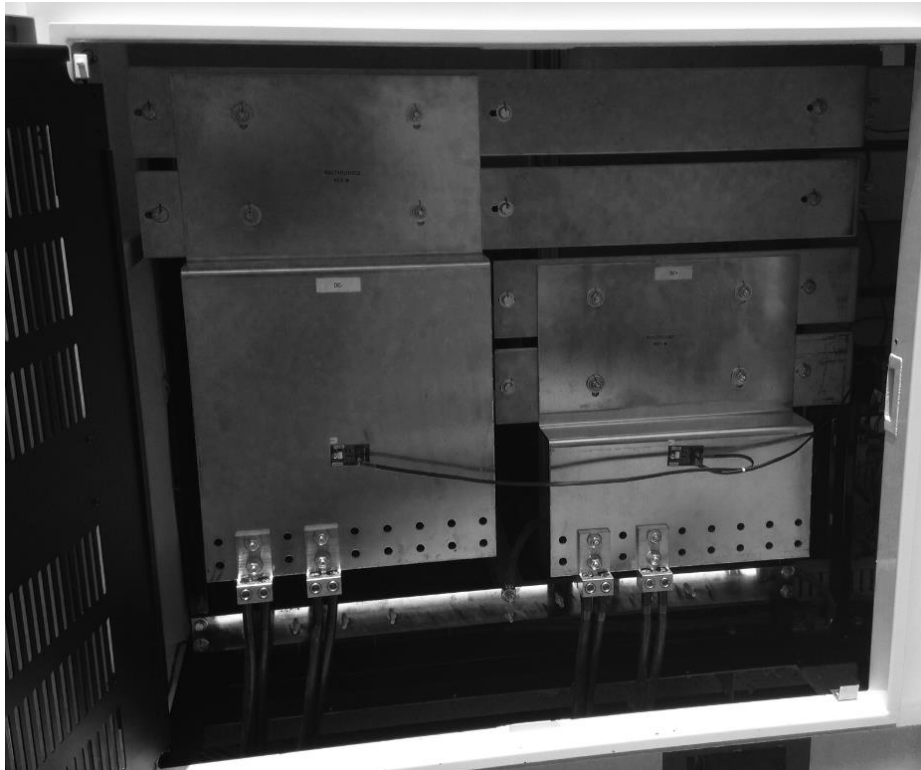
Figure 3-33: DC Input Locations (ACCESS DOORS #5(Right Side), #6(Left Side) and #7 (Inner Doors))
