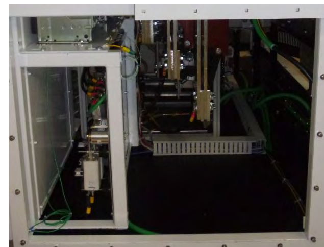
ACCESS COVER #4 / Strikesorbs, Current Transformers (CT-P1, CT-P2), Fuses (F2, 10F8, 10F9, 10F10, F11, F12, F17, F18, F19, 10F17, 10F18, 10F19, 10F20, 10F21), Power Meter (A4), Transformer (T1, T3, T4).
