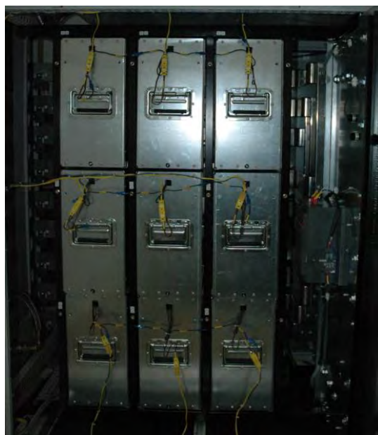
Figure 3-24: Filter Inductors (Behind Capacitor Door)
