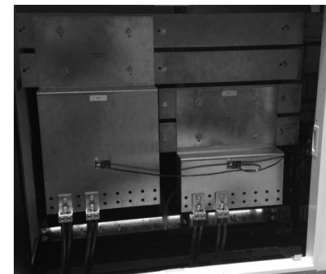
Figure 3-5: Battery Power Connections
