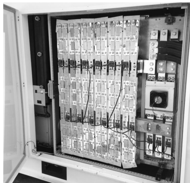
Figure 3-25: Filter Capacitors
