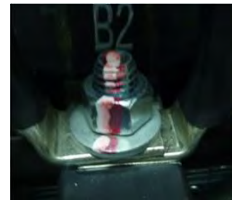
Example of marking bolted connection
