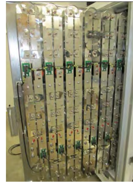
Figure 5-22c: GTB Filter Capacitor Panel
