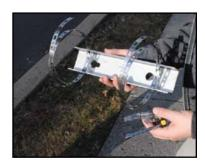
**Step #2** - For the most accurate results, the bracket should be installed so the Radar Recorder is facing traffic on a 45 degree angle. Once you have determined this position, wrap the bands around the pole and place the bracket.
