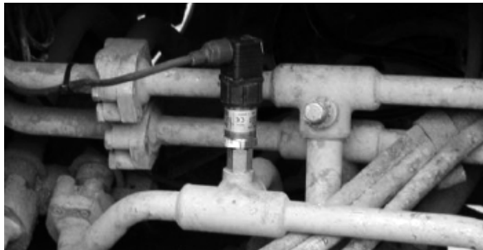
Figure 1-11. Sensor Mounted at Non-Recommended Angle
