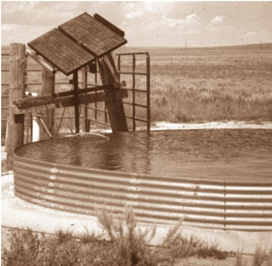
**Figure 3.** PV-powered pump systems often discharge to a storage tank to provide the daily water requirement even under low-light conditions. (Photo from National Renewable Energy Labs, 1997.)
