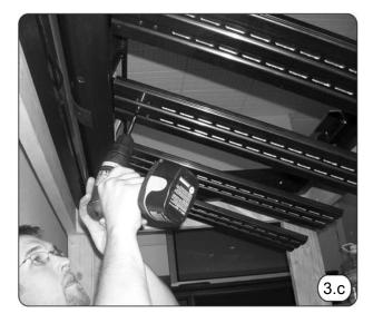
3.) Position TV sleeves over the TV mounting brackets and slide them into place (Figure:3.d).
