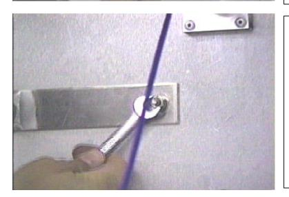
Carefully remove the four nuts and washers which hold the antenna to the mounting bracket, remove the antenna from the bracket, rotate the antenna 90 degrees, and refasten it to the mounting bracket. One Year Limited Warranty For products purchased using Solectek's U.S. & Canada MSRP Price List and installed in the United States or Canada. Effective August 1, 1999
