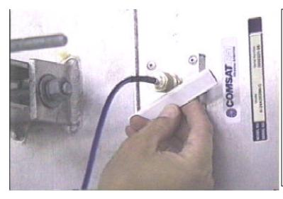
Use the sealer strips supplied with the antenna to seal the connector. Peel the paper backing from the strips and stretch the material while winding it around the connector. Be sure to cover all exposed metal. This large (Ntype) connector will probably require two strips for a proper, weather tight seal. Use your fingers to form the sealant against the connector for a good seal.
