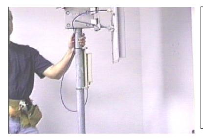
Use Ty-Wraps or other fastening material to hold the antenna cables securely against the mast.
