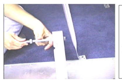
Locate the "V" cut in the mounting arm. The "V" cut will grip the mast when the antenna is installed. Install the long mast-clamp bolts as shown. Use one nut to securely mount the long bolts to the mounting arm by turning the nut all the way to the end of the thread so it securely holds the bolt in the mounting arm.
