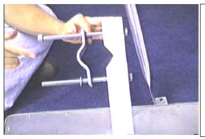
Install the mast clamp strap as shown. The strap makes a channel with the "V" cut in the mounting arm. The mast pipe will pass through this channel. Do not tighten the nuts.
