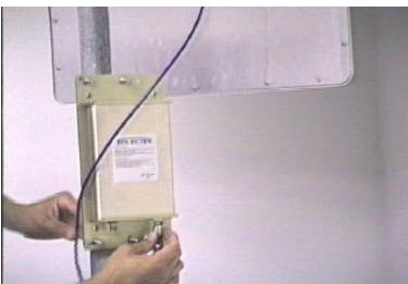
Attach the antenna-to-ODU cable to the ODU (Outdoor Unit). Finger tighten the connector. No threads should be visible when the connector is properly tightened and seated.
