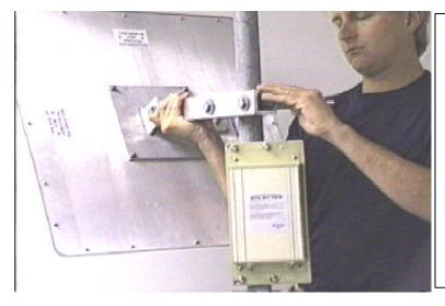
Install the antenna and preassembled bracket on the mast. Tighten the two nuts so the antenna is held securely to the mast. Do not overtighten to the point where the mounting strap is deformed. These nuts will be loosened later to swing the antenna on the mast to adjust the azimuth during antenna alignment.
