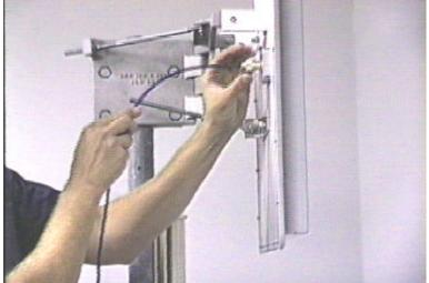
Install the supplied antenna to ODU cable. The cable cannot be installed backwards, as the connectors are different on each end.
