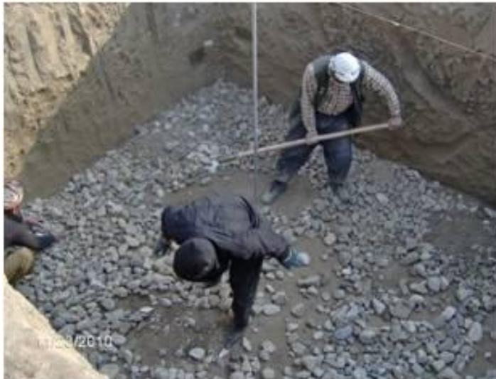
Photo 7.1: Cobbles and Gravel Placed on Compacted Earth Floor.
