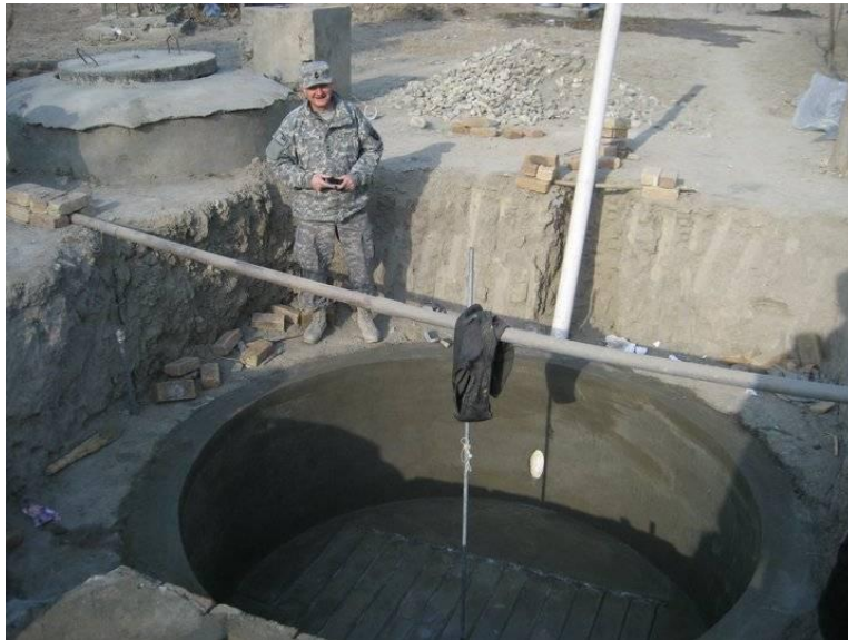
Photo 7.4: Inlet Pipe Installed in Digester.
