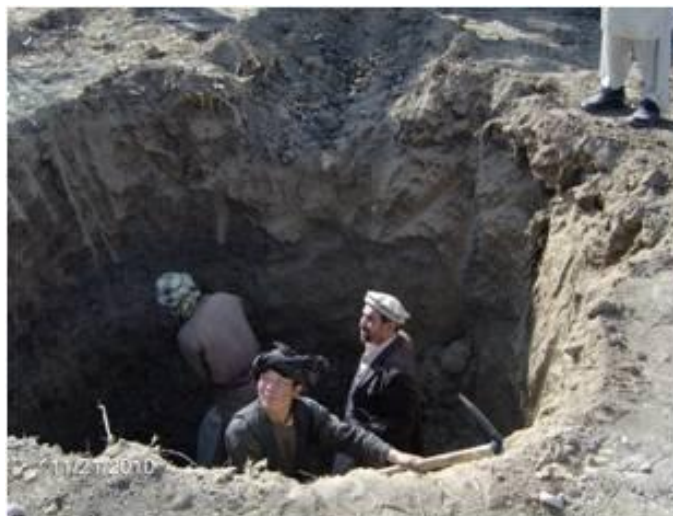
Photo 6.2: Excavation for Digester. Mechanical or Manual Excavation is Practical.
