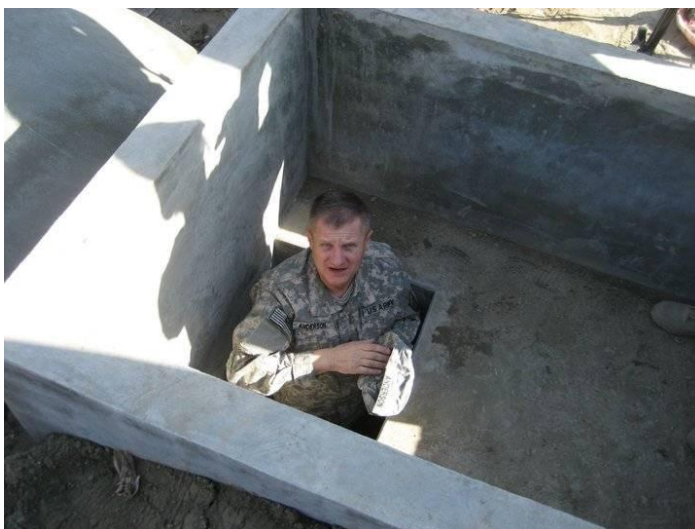
Photo 9.4: Manhole Inspection of Complete Outlet Chamber.
