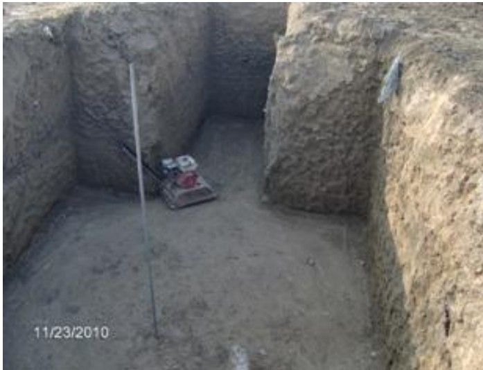
Photo 6.3: Earth Base of Excavation is Compacted.
