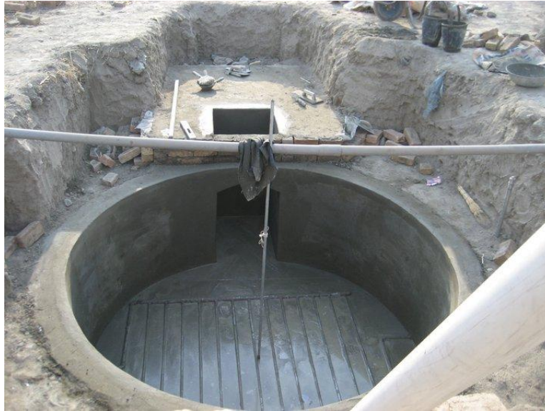
Photo 7.5: View of Manhole in Main Digester.
