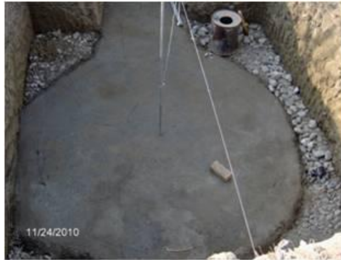
Photo 7.2: Concrete Foundation for Digester. Center Guide Pipe and Horizontal Cord.
