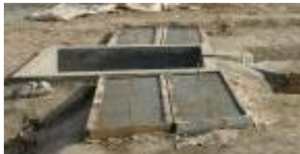
Photo 9.2: Outlet Chamber Slabs in Casts.
