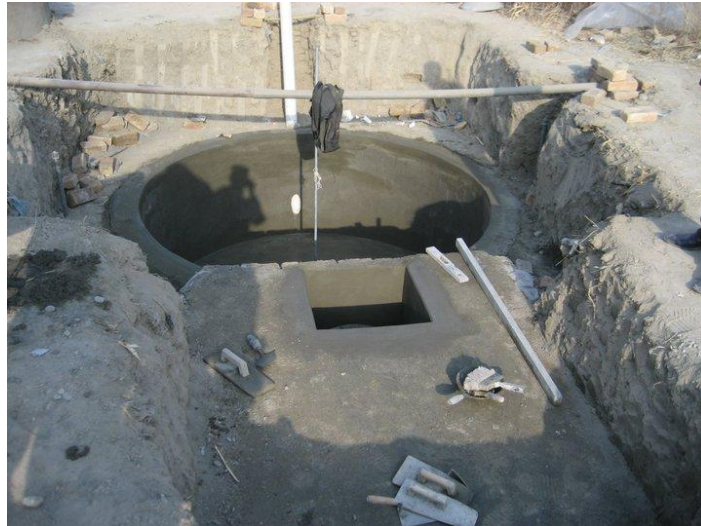
Photo 9.1: Outlet Chamber Foundation of Brick with Manhole Adjacent to Digester.
