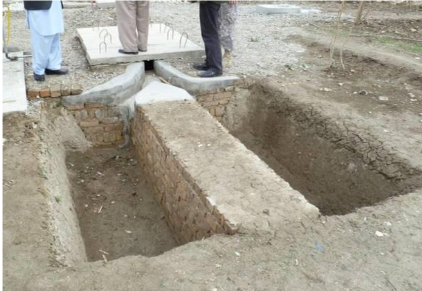
Photo 12.1: Compost Pits with Brick Walls for Stability
