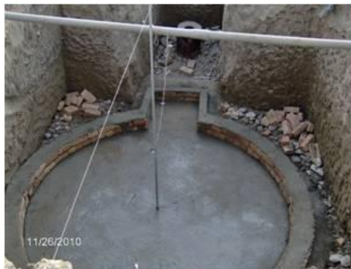
Photo 7.3: First Two Courses of Bricks Placed on Top of Foundation.
