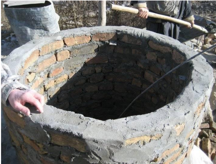
Photo 10.1: Inlet Tank During Masonry Construction.
