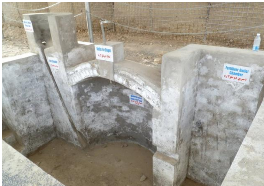
Photo 2.1: Scale Model of 4 Cubic-Meter Biogas Plant for Training (Camp Nathan Smith, Kandahar, Afghanistan)
