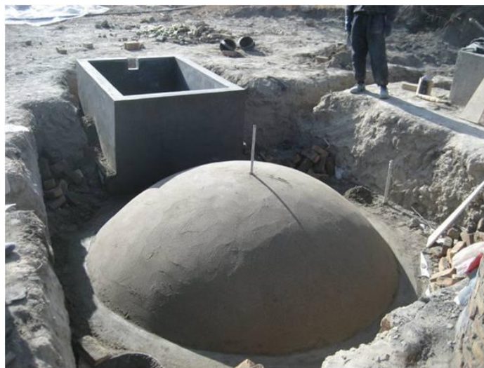
Photo 8.4: Earth Mould with Sand Layer Before Placing Cast.
