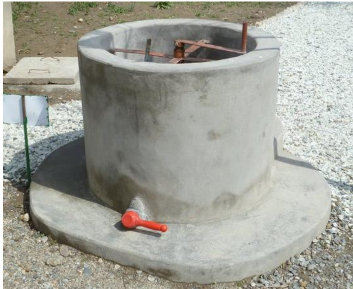
Photo 10.2: Complete Inlet Tank with Mixer and Ball Valve on Inlet Tube.
