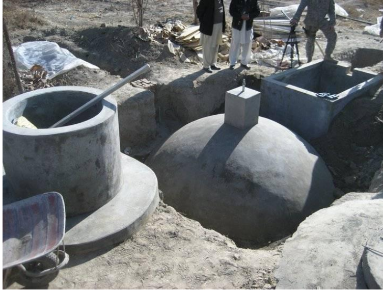
Photo 8.6: Completed Dome with Turret.
