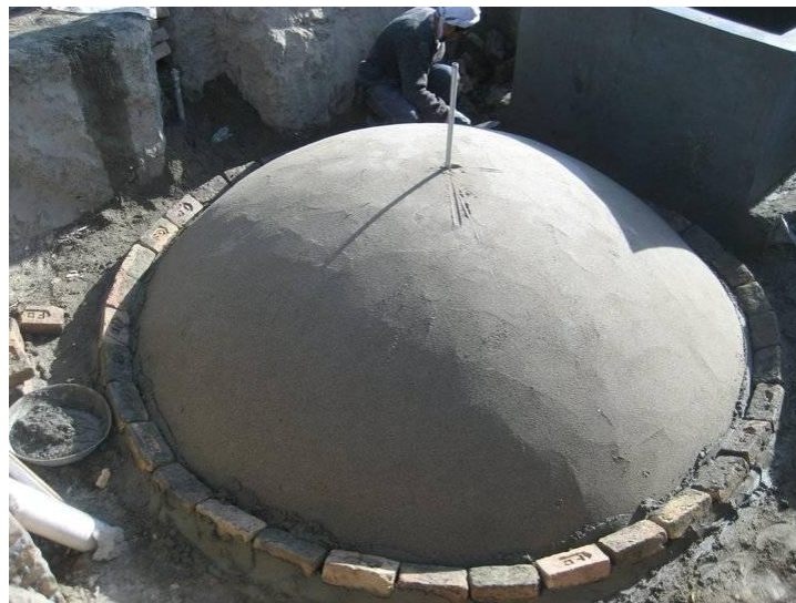
Photo 8.5: Earth Mould with Sand Layer Before Placing Dome (Brick).
