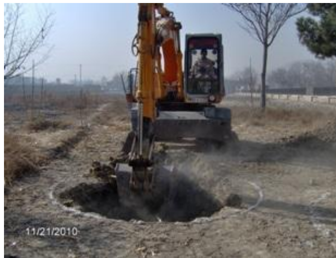
Photo 6.1: Excavation for Digester. Mechanical or Manual Excavation is Practical.
