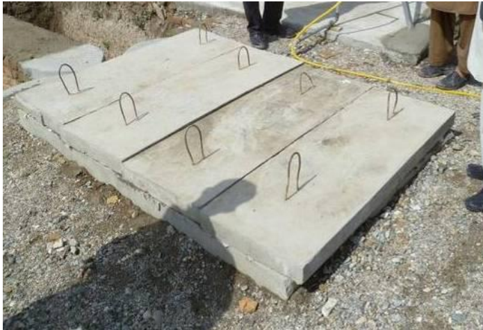
Photo 9.3: Slabs in Place on Outlet Chamber.
