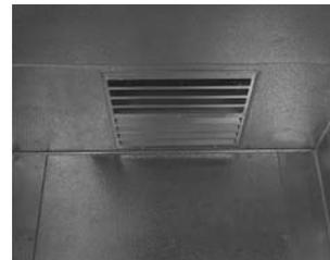
The PRO<sup>3</sup> Top Mount evaporator grill sits flush in a standard 4" thick ceiling panel.
