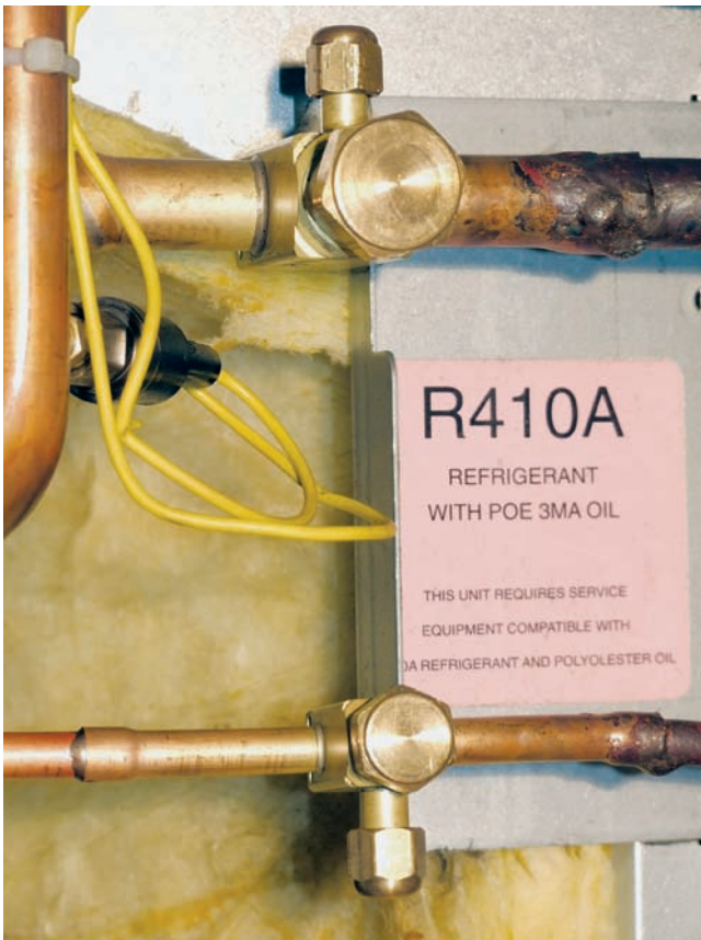
Figure 25-4 Residential split system installation valves
