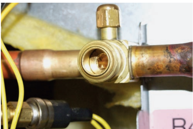
Figure 25-18 The condensing unit is shipped with the valve closed to hold in the system refrigerant
