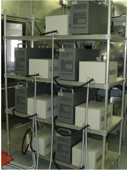
Figure 2-5. The power rack houses a converter and transformer for each lamp assembly on the simulator. Photo courtesy of Ben Erickson.
