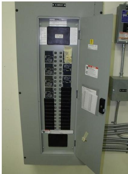
Figure 2-4. Power to each lamp can be individually turned on or off at the main power box. Photo courtesy of Ben Erickson.
