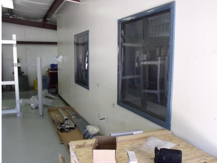
Figure 2-13. The windows into the control room are protected by removable plexiglass sheets. Photo courtesy of Ben Erickson.
