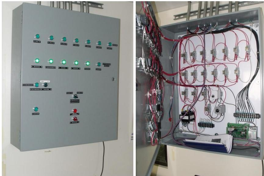
Figure 2-16. The safety panel which alerts the users to open doors and allows for power to be supplied to the simulator if all interlocks are active. Photos courtesy of Ben Erickson.
