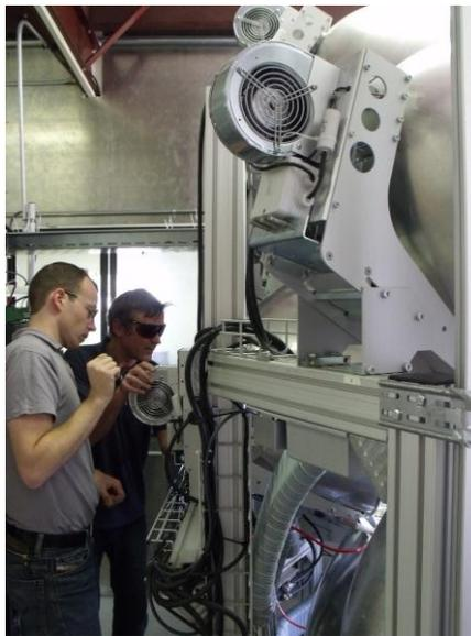
Figure 2-12. Installation of the power and cooling systems. Photo courtesy of Ben Erickson.
