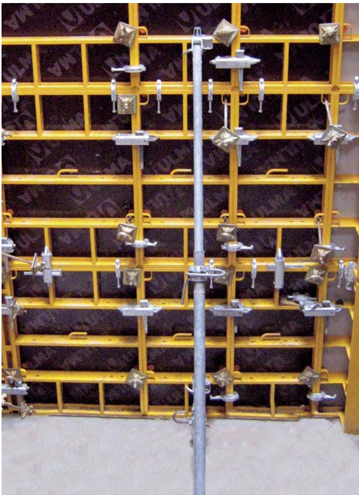
▲ Gangs stabilized by Push-pull prop
