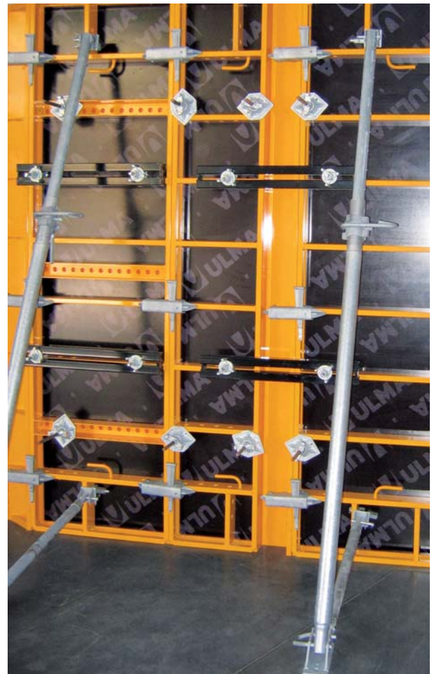
▲ Push-pull prop fixed to a horizontal rib
