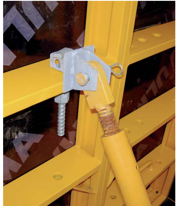
▲ Push-pull prop fixed to a horizontal rib
