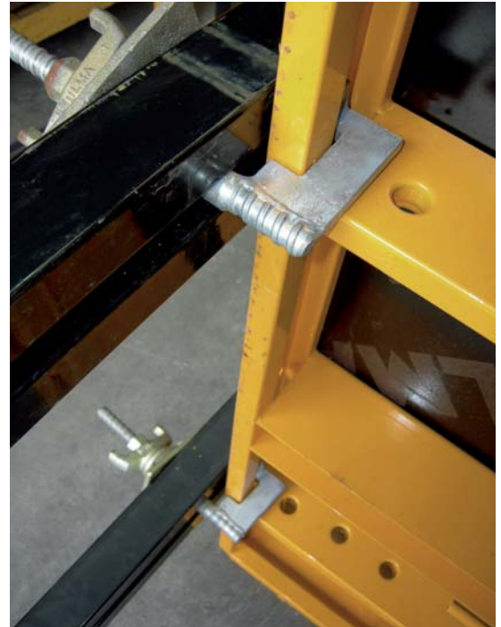
▲ Fixing the Waler to the Panel using Bulkhead Hooks
