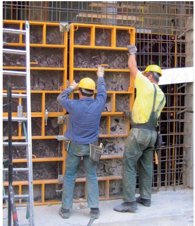
▲ The NEVI Modular Formwork lightweight allows handset assembly
