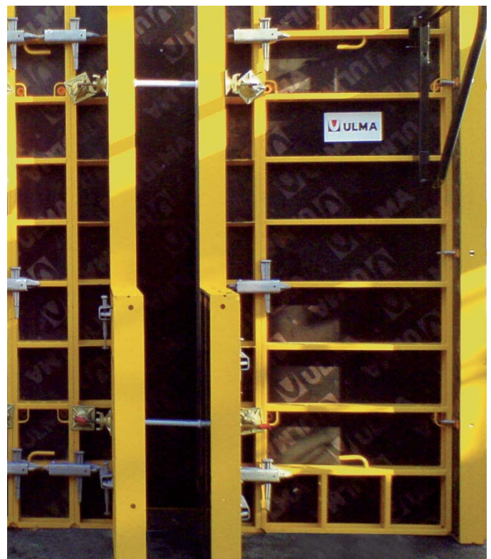
▲ Being protected by plastic tube, the rods are reusable
