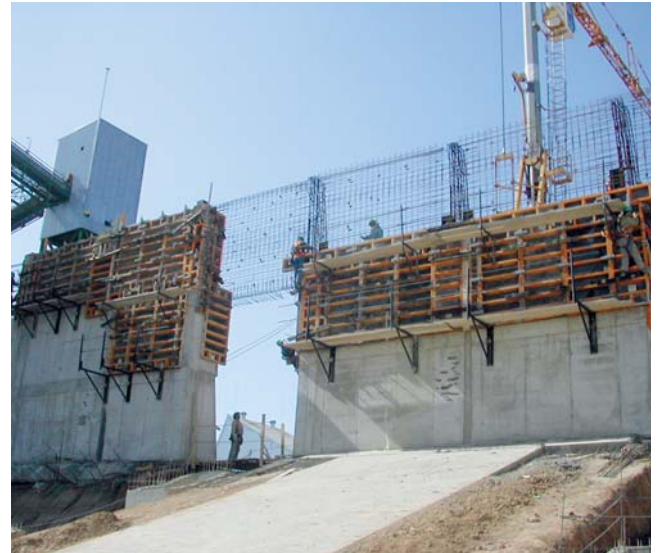
▲ Climbing Bracket support system
