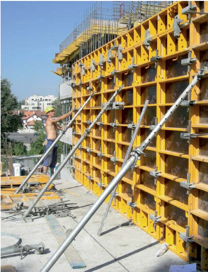
▲ Gallery inside formwork stabilized to the ground
