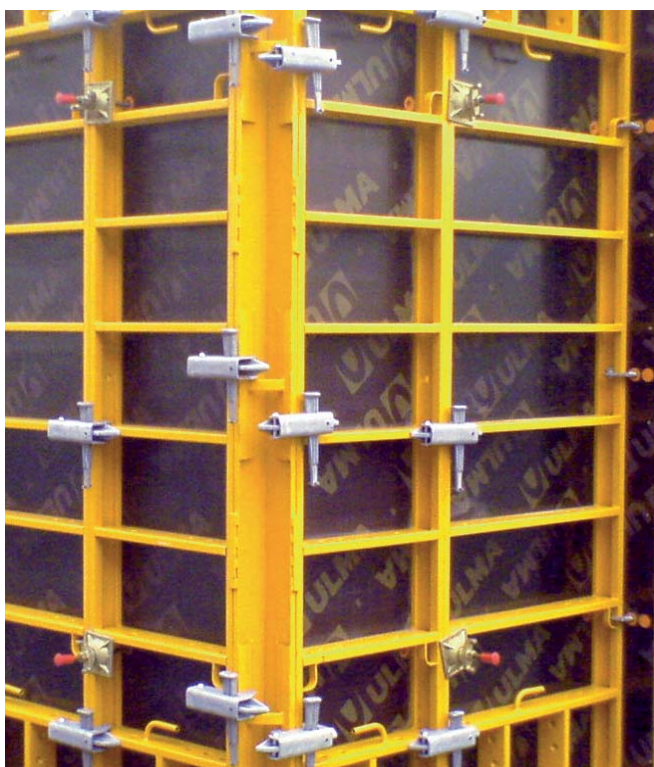
▲ Panel-Outside Corner joint with Adjustable Clamps
