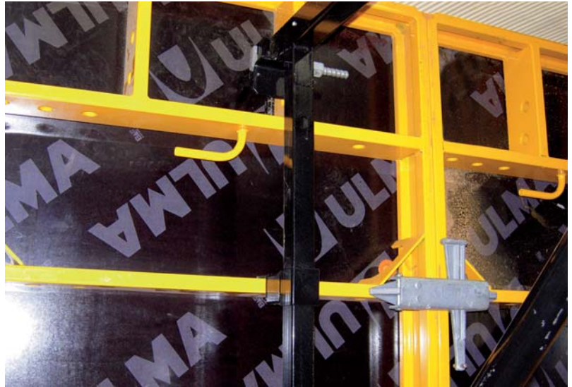
▲ Detail: fixed to a vertical rib
