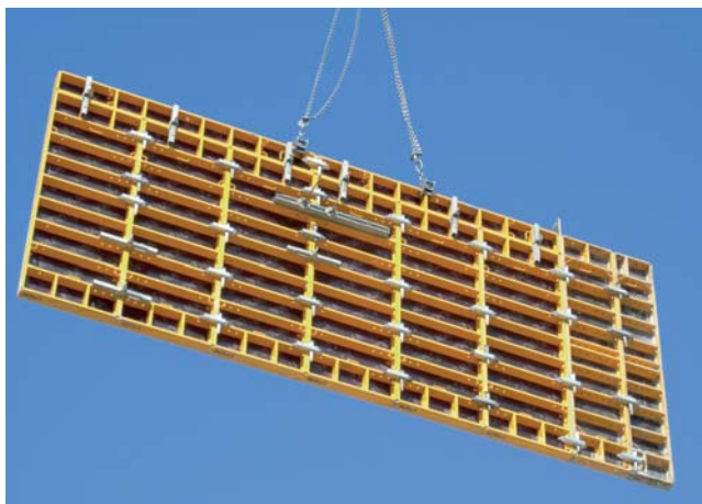
▲ It is recommended to use two lifting hooks when lifting
