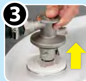
3 Pull Coupler up & Remove
