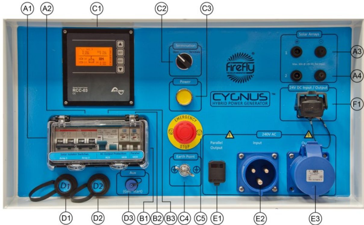
Fig. 1 - Cygnus Control Panel Component Reference
