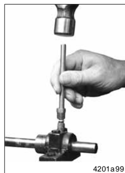
Fig. 2-2 Installation of Zerk-Locks with staking tool
