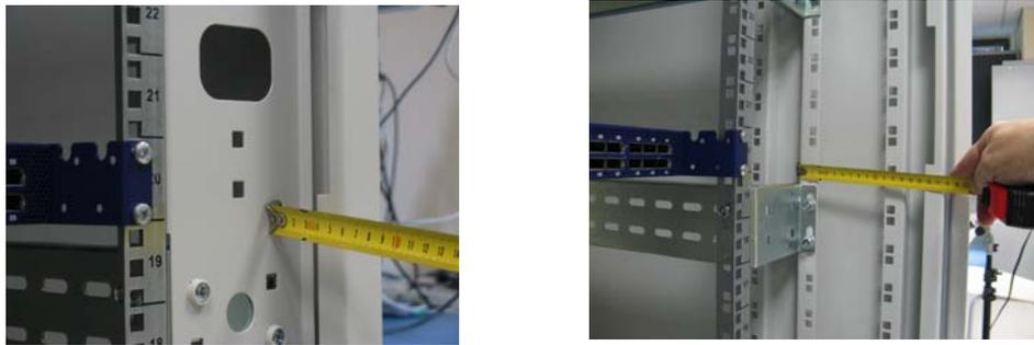
The distance between the rack and the door can be as little as 4 cm on one side of the rack and as much as 18 cm on the other side of the rack. Keep in mind that there can be as many as 36 cables connected to the switch.
