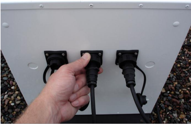
Figure 39: Connect Solar Cells to Battery Enclosure Box
