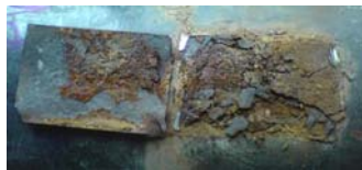
Fig. 5 Corrosion present under an air tank label
