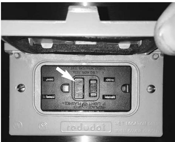
**Figure 4-2.** Reset Button on GFCI Outlet
