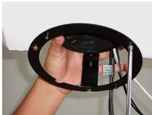
Make sure the safety hook is secured and follow the clockwise direction to attach the Speed Dome main body into the embedded ring.
