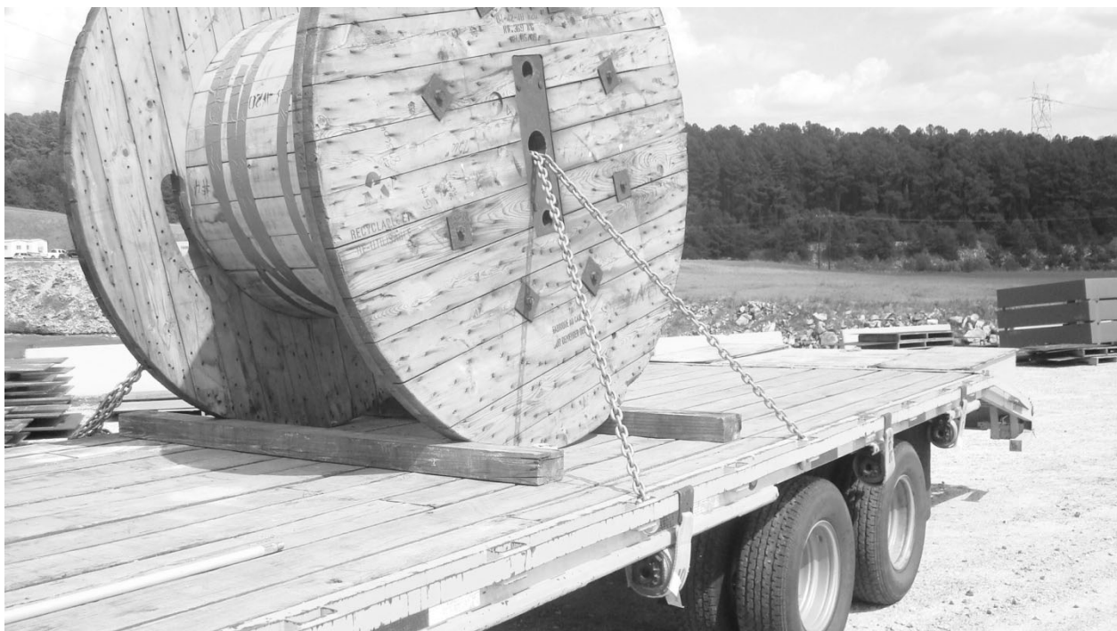
Figure 8-1 Correctly Secured Reel Ready for Transport
