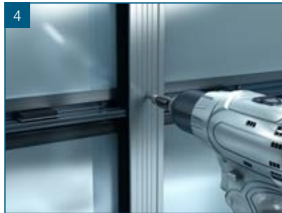
4.1. Fix vertical pressure plates using correct screws with a torque of 3.2 nm.
