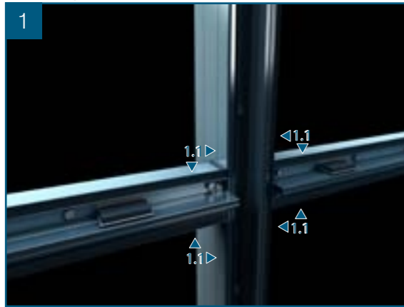
1.1. Before the fitting of glass, it is recommended that petroleum jelly is applied to both the front and rear gaskets. This allows for easier positioning of the glass in the curtain wall opening as well as allows glass to seat better onto the gaskets.
