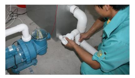
Fig.C9-1: Pipe between Circulating Pump and Mechanical Belt Filter.
