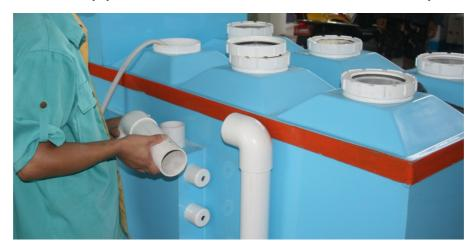
Fig.C11: Connect the outlet pipe to your culture tank.\*
