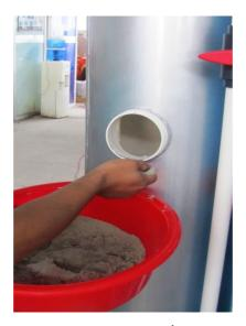
Fig.C6: Fill the sand into the bioreactor. (Through the side opening)
