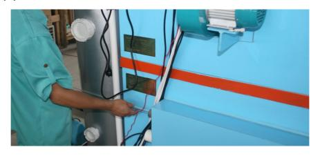
Fig.W3-1: Installation of UV lamp into the system
