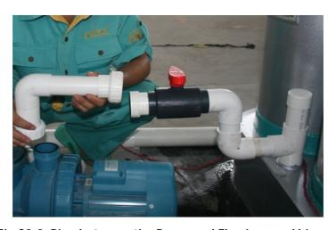
Fig.C8-2: Pipe between the Pump and Flowing-sand bioreactor.
