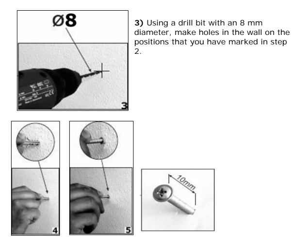
4) Insert rawl plugs into all of the holes that you have drilled.
