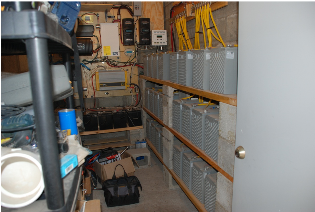
Right side - Twenty four AGM sealed batteries (each 12V@120AH)
