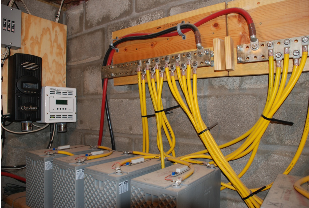
Notice the small battery balancer circuit boards wired across each battery
