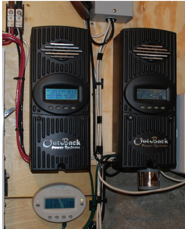
Two Mx-60 Synchronized Chargers from Outbackpower.com
