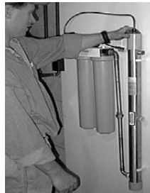
Install UV unit
