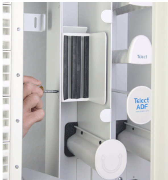
Figure 9 - Installing Parking Lots
