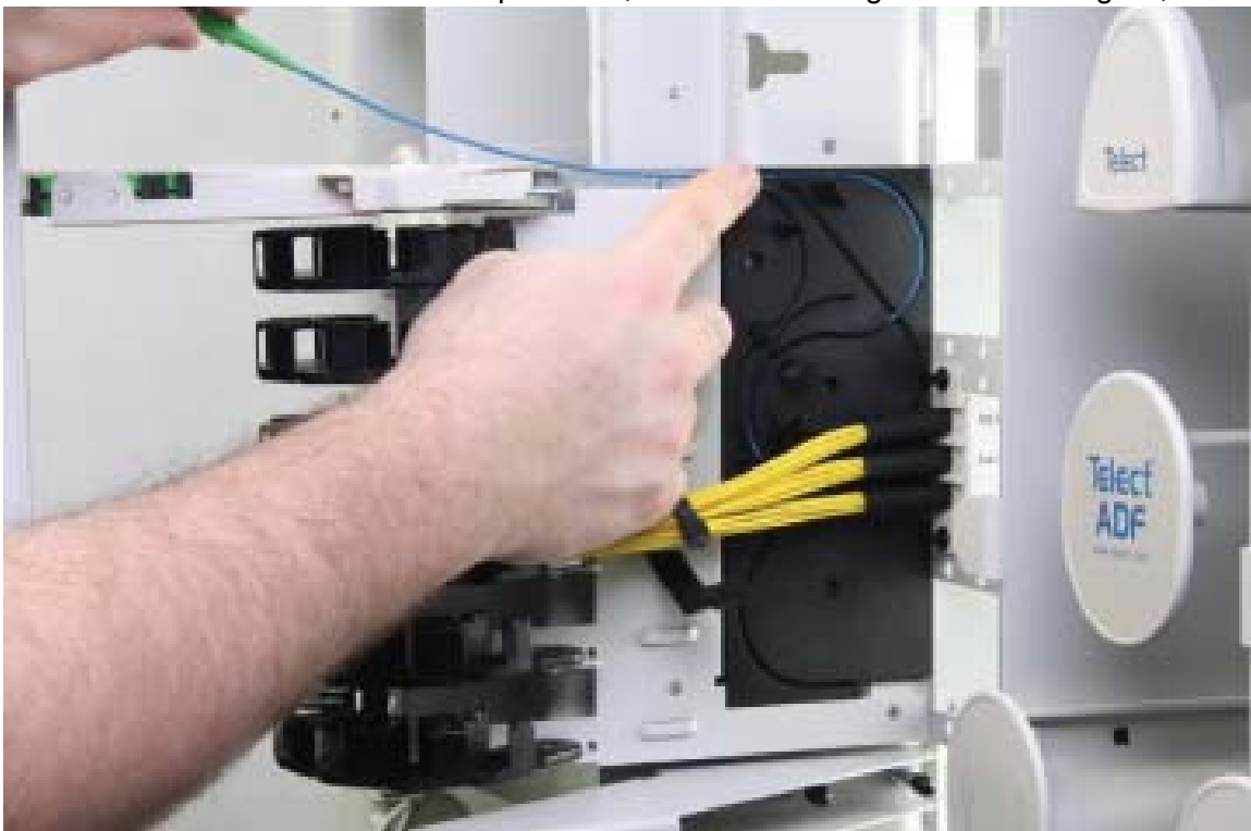
Figure 33 - Routing the Wires for the Third and Fourth Positions
