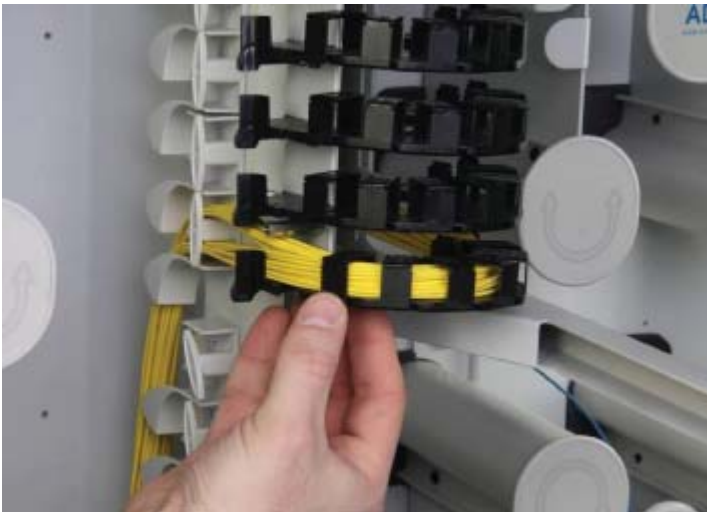
Figure 23 - Latching the Link Chain
