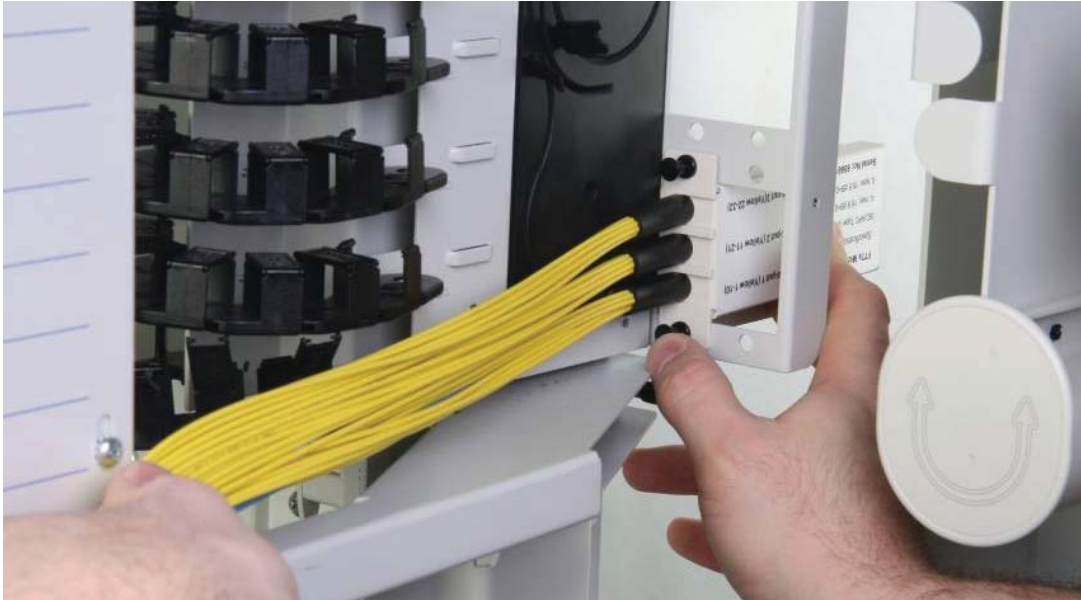
Figure 16 - Installing the Splitter Modules
