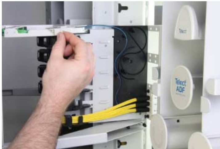
Figure 31 - Closing the Routing Area
