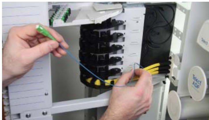
Figure 27 - Routing the Input Fiber
