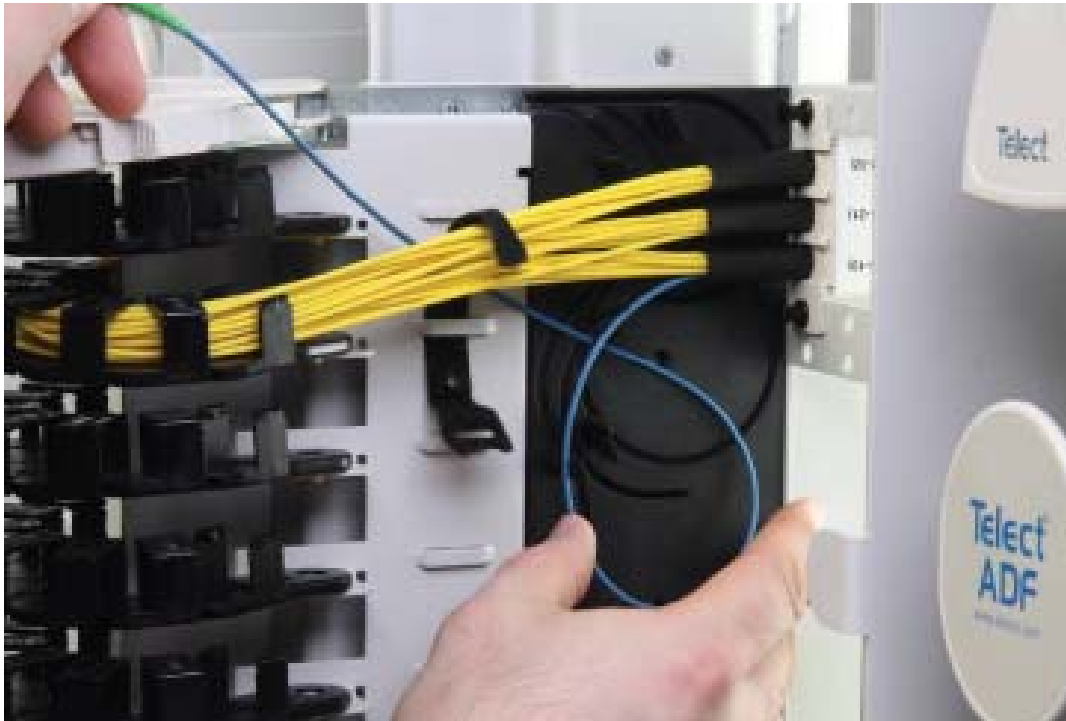
Figure 34 - Routing the Wires for the Fifth and Sixth Positions
