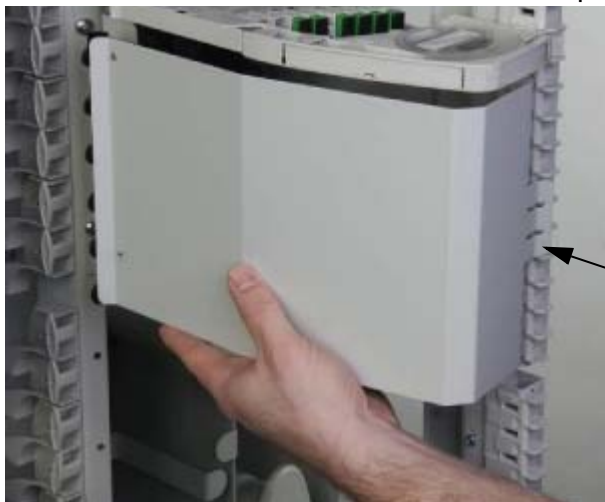
Figure 11 - Lifting the Cover off the Pegs
