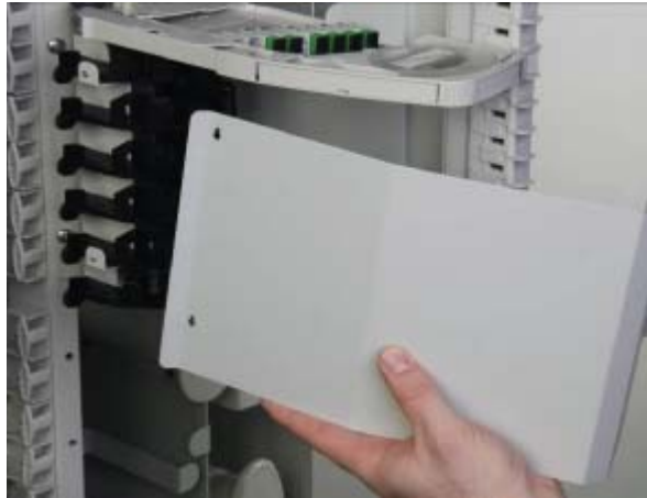
Figure 12 - Lifting off the Cover, continued
