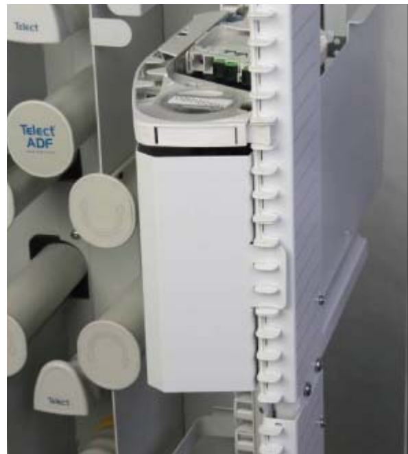
Figure 6 - Snapping the Tray and Cover into Position
