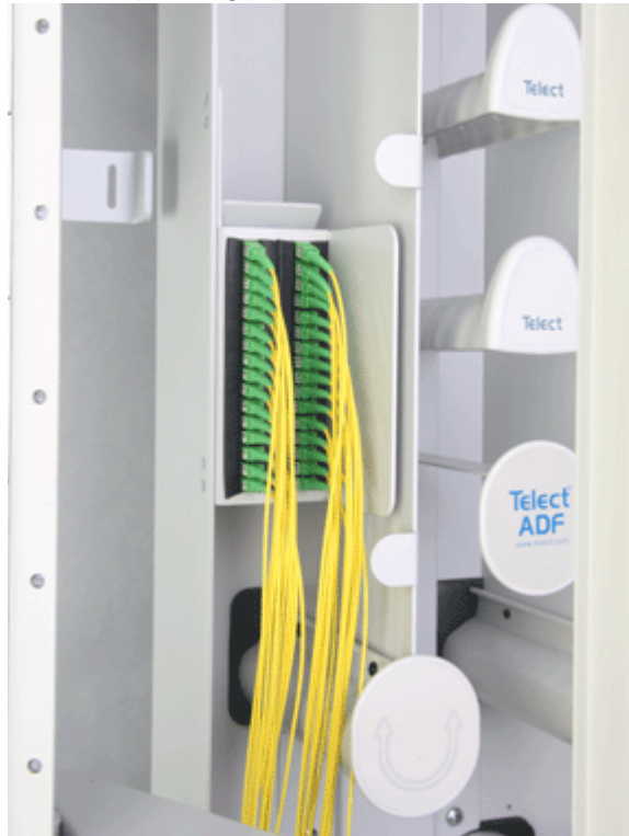
Figure 26 - Installing Fiber Connectors
