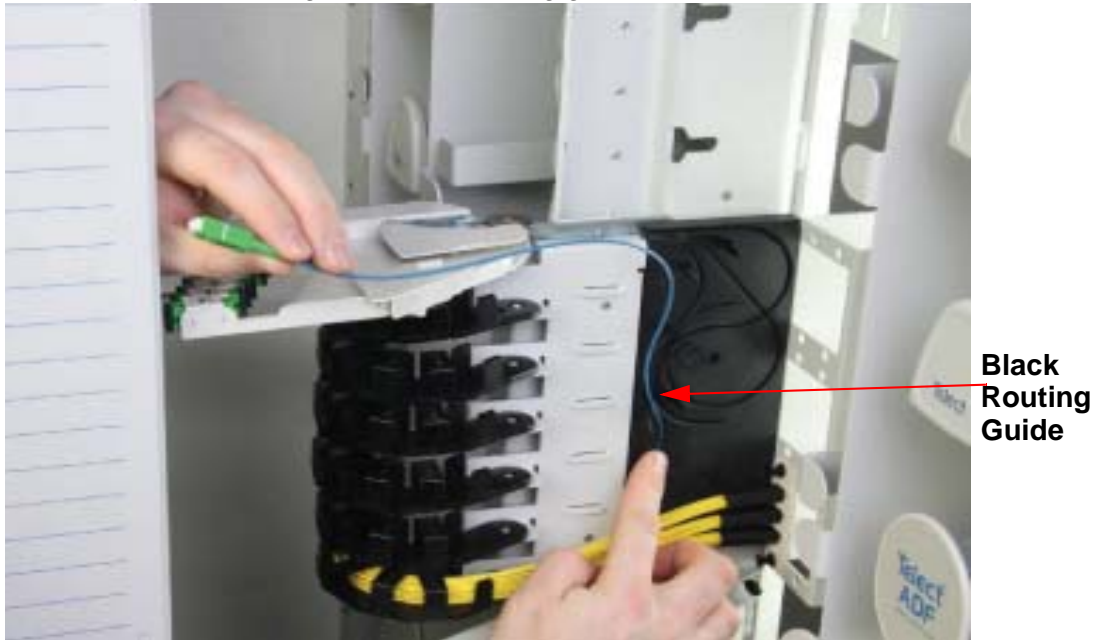
Figure 28 - Routing the Input Line
