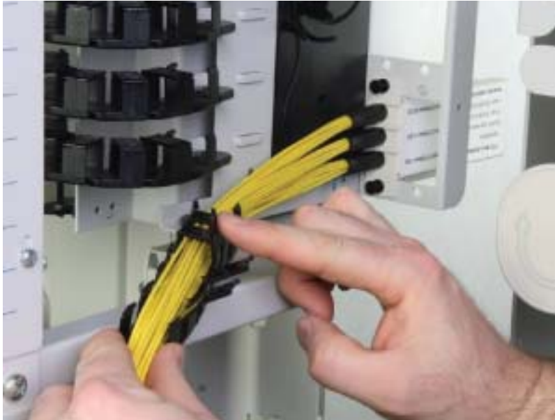
Figure 18 - Closing the Link Lids
