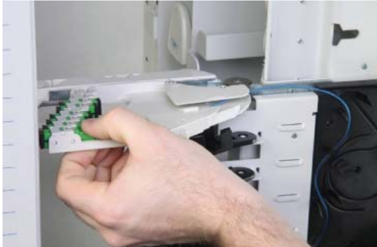
Figure 30 - Inserting the Connector, continued
