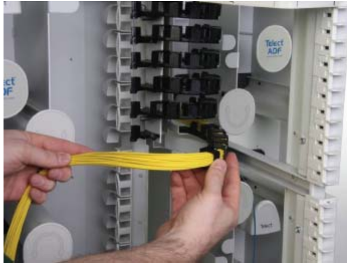
Figure 20 - Bring in Cables
