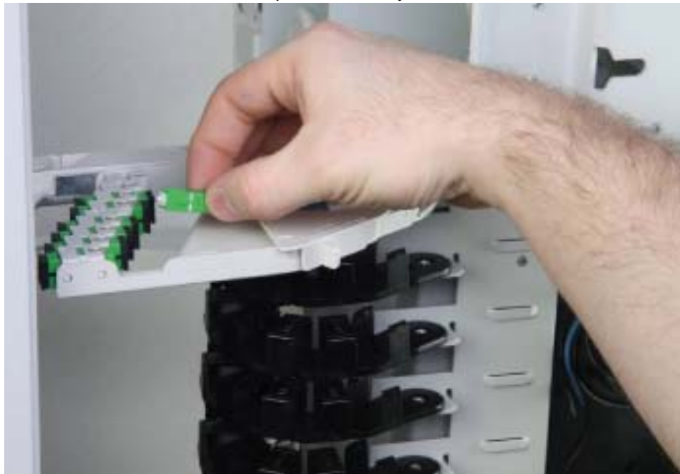
Figure 29 - Inserting the Connector
