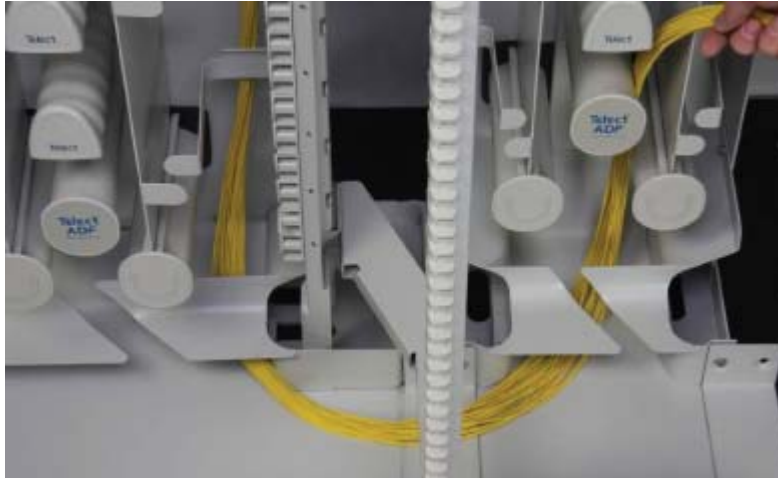
Figure 24 - Routing the Fiber Cable
