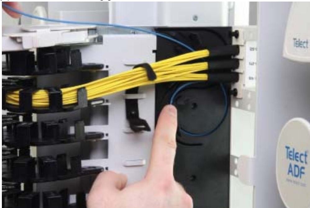
Figure 35 - Inserting Fiber into the Routing Guide
