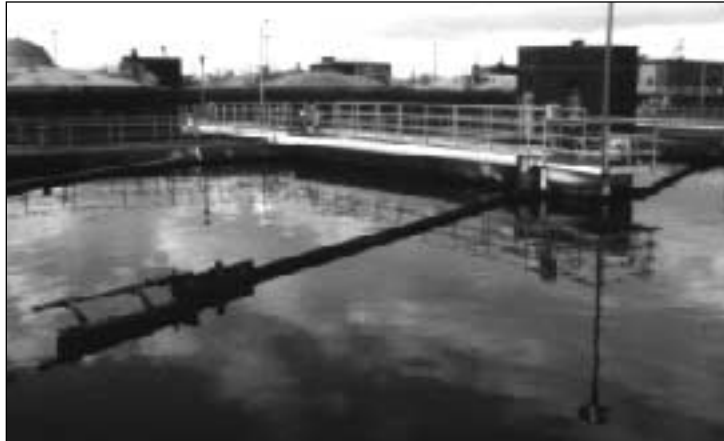
Wastewater treatment facility
