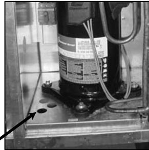
Piping to gas valve inlet must be completed in field.
