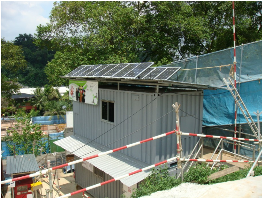
1.6kWp photovoltaic powered modules
