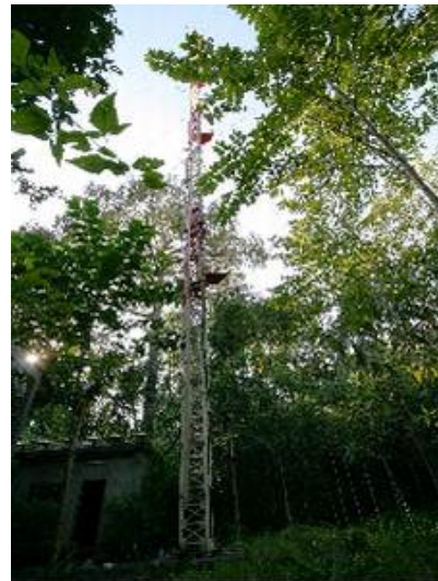
Photo 1.2-3 “Ladder tower” with a ladder-like part for easy access. (Kampong Thom Province, Cambodia. Photograph: courtesy of Shimizu Akira)
