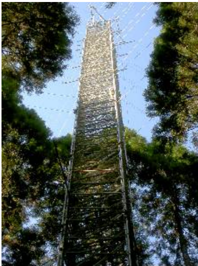
Photo 1.2-2 “Scaffolding tower” with access stairs. (Kahoku Experimental Watershed)
