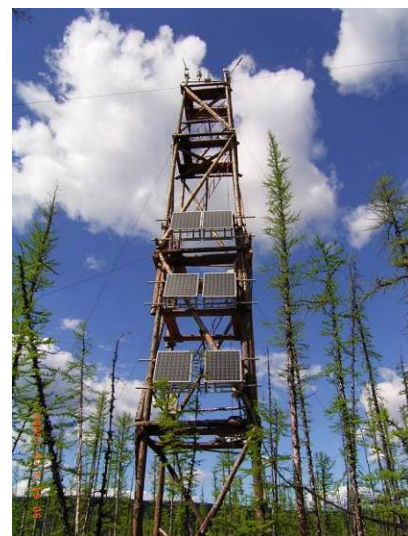
Photo 1.2-8 A flux observation tower using solar cells. (Tura, Russia)
