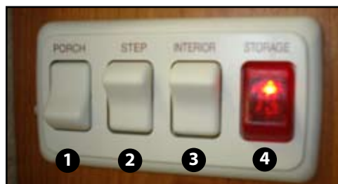
ENTRY SWITCH PANEL
