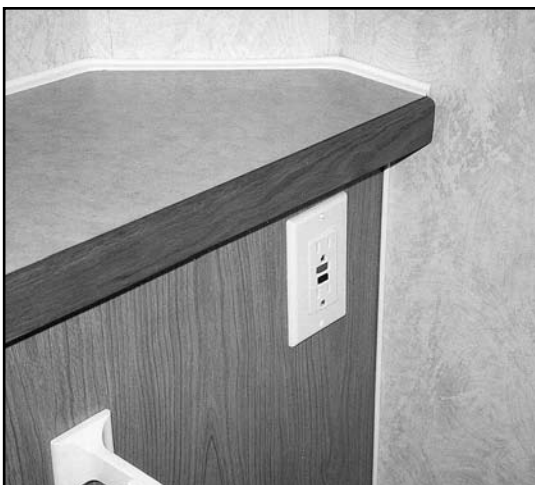
GFCI OUTLET (TYPICAL)
