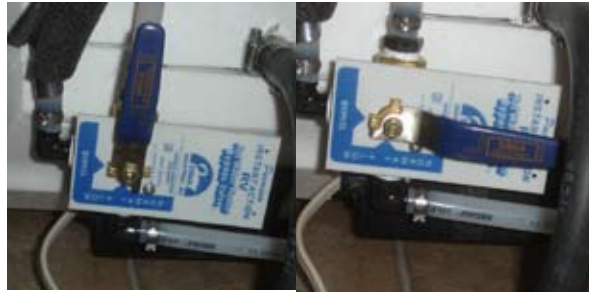
1. NORMAL POSITION 2. BYPASS POSITION
