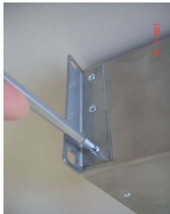
Fig. 3: Rack angles assembly
