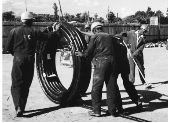
Figure 4: Uncoiling Pipe
