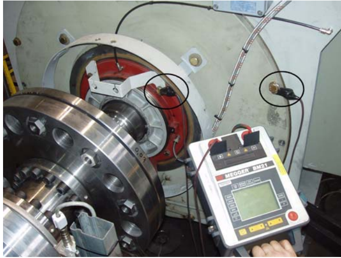
Figure 7-4 Measuring the insulation resistance of a roller bearing
