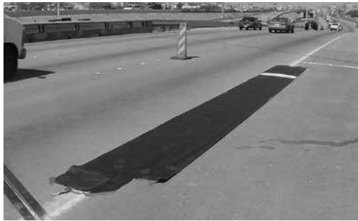
Figure 5—Tar Paper Layout for a Test Spray
