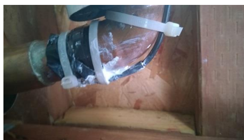
FIGURE 6. GROUND LOOP TEMPERATURE SENSOR (INSULATION REMOVED TO SHOW MOUNTING)
