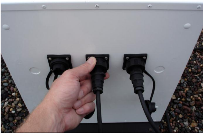
Figure 47: Connect Solar Cells to Battery Enclosure Box
