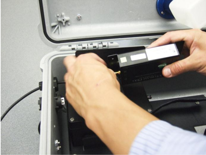
Figure 12: Attach Antenna and Cable to Radio Modem
