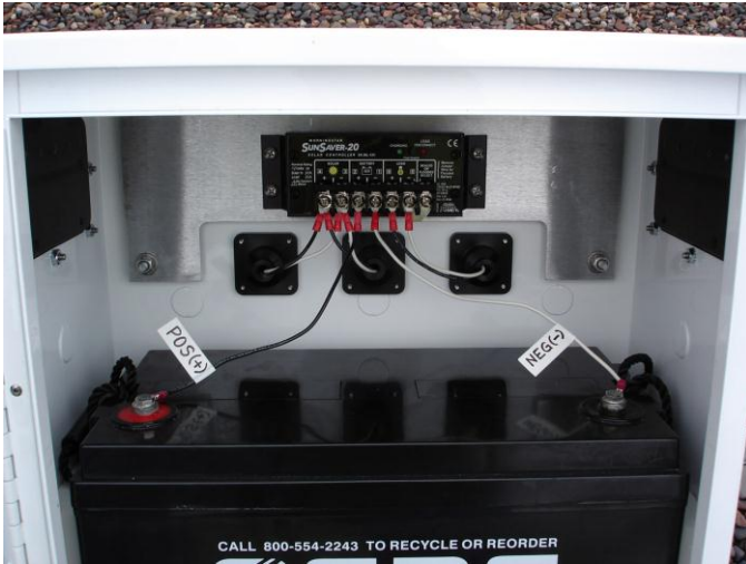
Figure 39: Install the Solar Battery and Connect to Controller
