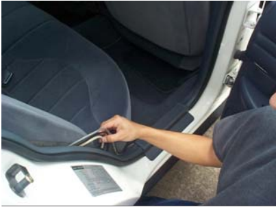
View of DB-25 and power cables coming from trunk, positioned behind the rear passenger side seat, heading toward front passenger seat. Note: cables go under carpet.
