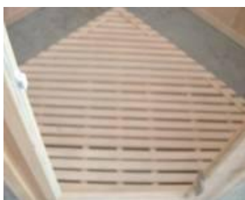
FIG-9 place the floor board
