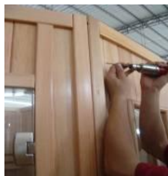
FIG-8 lock the screw on the right of the front board
