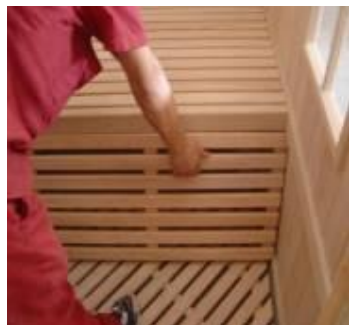
FIG-13 Assembling right short baffle
