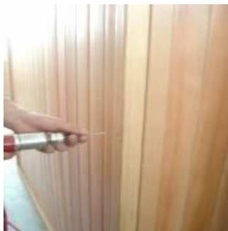
FIG-5 Lock the screw tight
