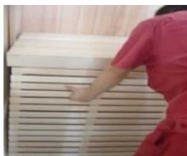
FIG-12 Assemble the left long sitting baffle
