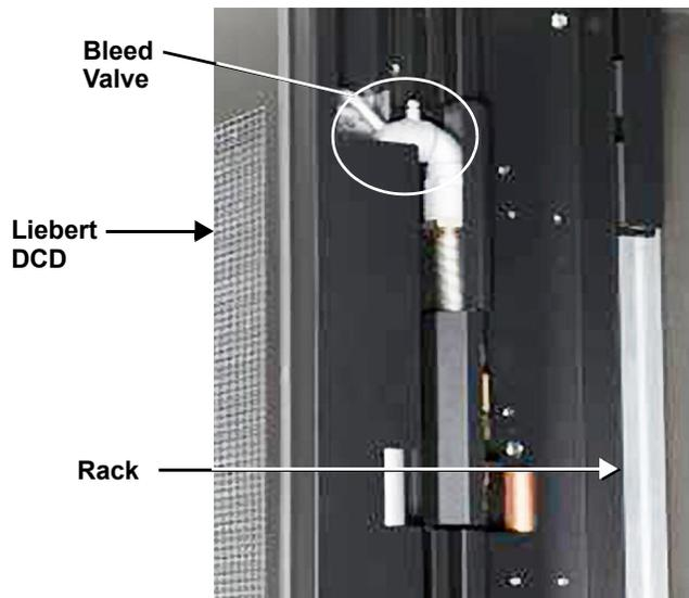
**Figure 24** Liebert® XDK-W™ bleed valve
