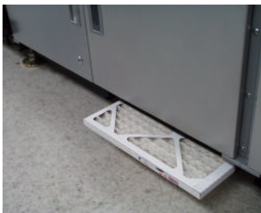
Figure 5-15 Purolator Hi-40 System Filters
