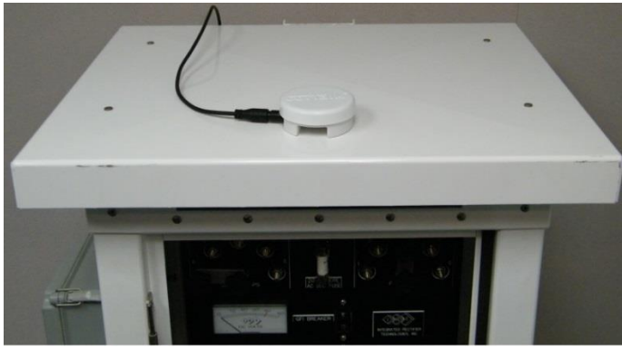
Figure 19 Mounted On Top of a Rectifier Cabinet (uGI1 LCD Display Facing Down)
