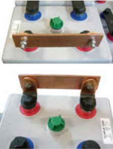
Fig. 5-18: Installing the end terminals (connection plates)
