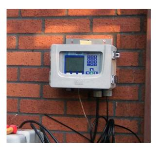
Figure 3-13 Signature Flow Meter mounted on wall
