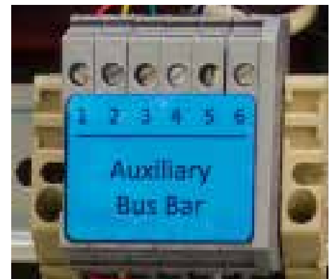
Fig. 7 - Auxiliary Bus Bar
