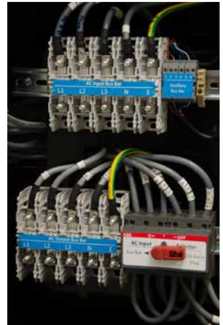
AC & Aux. Bus Bar Connections, Input Selector Switch
