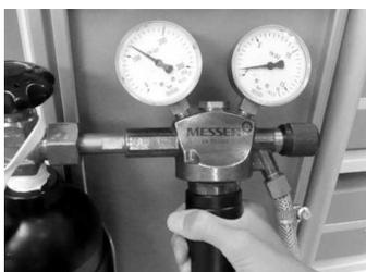
Open the main valve of the gas cylinder and set the secondary pressure to 1 bar
