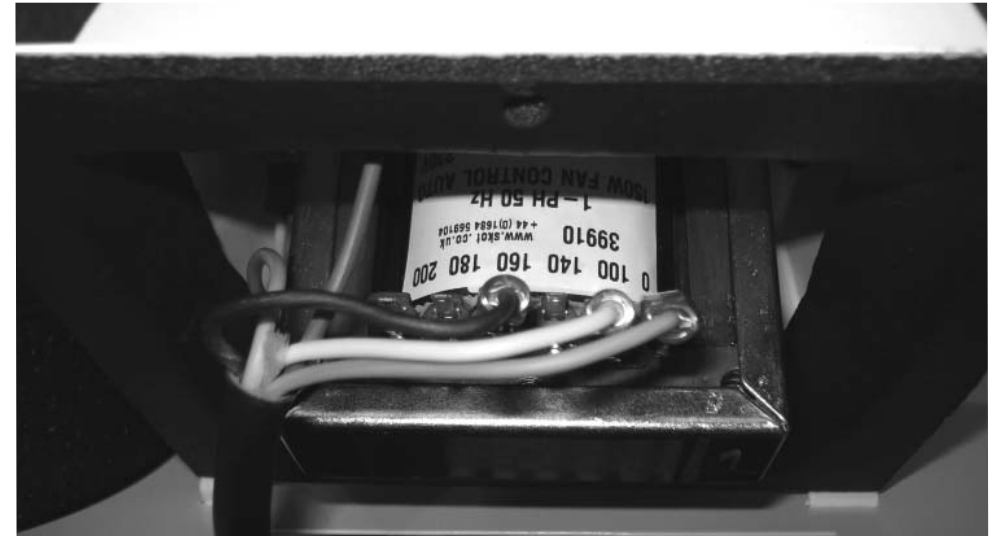
WHITE wire continuous rate, BLACK wire boost rate. Do not reposition the BROWN or BLUE wire.
