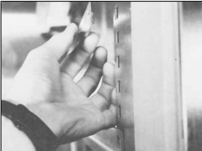
Figure 2-9 Installing Stainless Steel Angle Type Pan Slides
