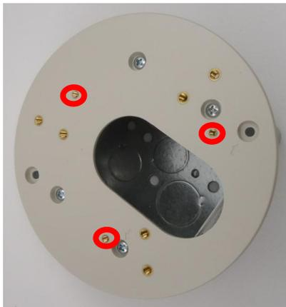
Connect cables through the hole on PMAX-0803 accessory.
